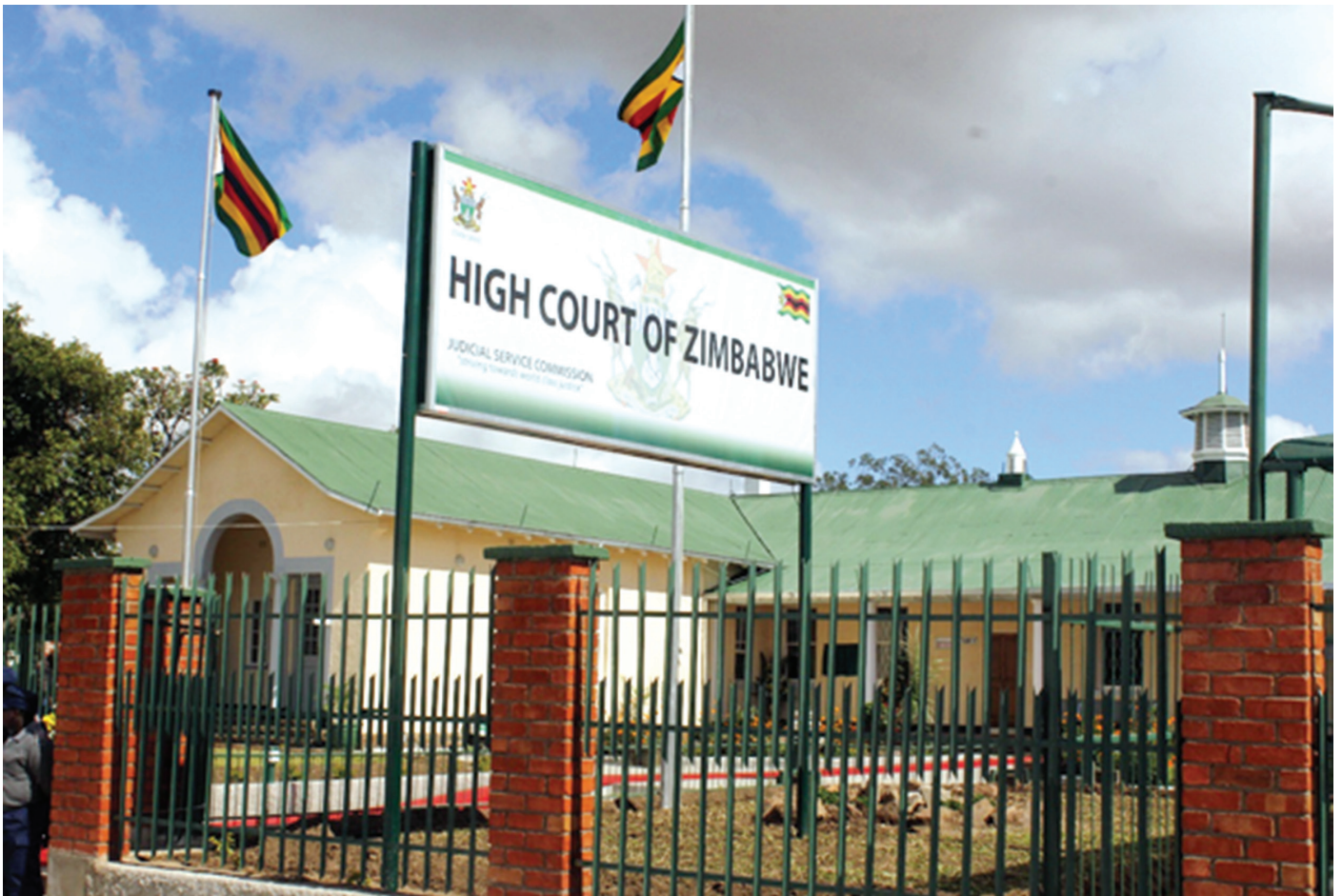
The newly opened Masvingo High Court building
