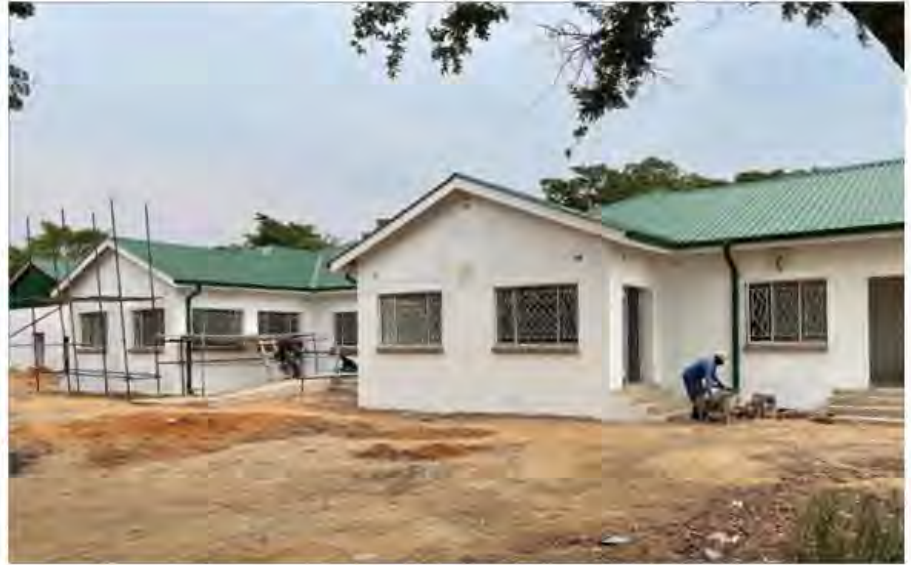
Epworth Magistrates' Court under construction
